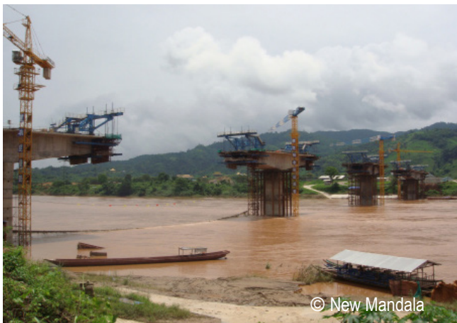
China has heavily invested in bridges and pipelines throughout the Mekong region.
