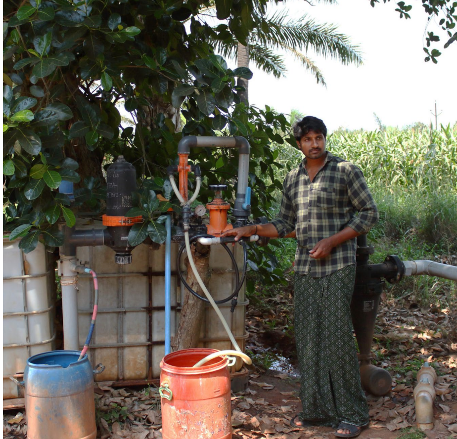
L. Rama Rao's son Pradeep looks after their farm's drip irrigation system, which can also be used to deliver fertiliser to their oil palms (Image: Kevin Samuel / China Dialogue)
